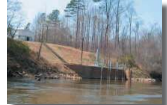
Johnston County water treatment plant on the Neuse River.
