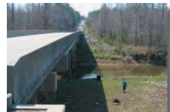
Bridge at Fire Dept. Road.
