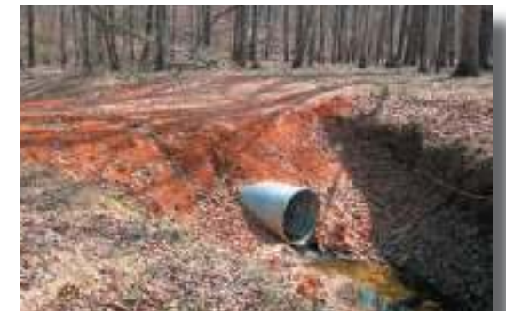
New subdivision construction along the river.
