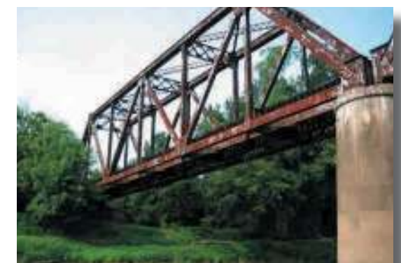
Railroad bridge near US 70.
