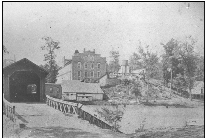
Photo 3: Worthville Covered Bridge looking south toward factory. Photo courtesy of Mac Whatley.
