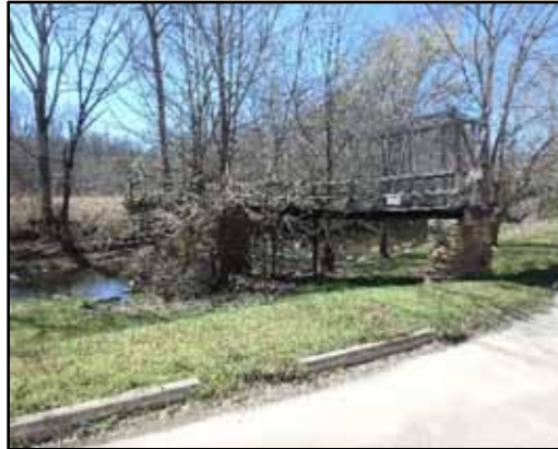
P2 – Old bridge structure at Cedar Falls
