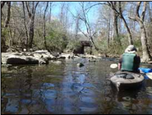
P5 – Hasketts Creek with WOW Rd. bridge in the background
