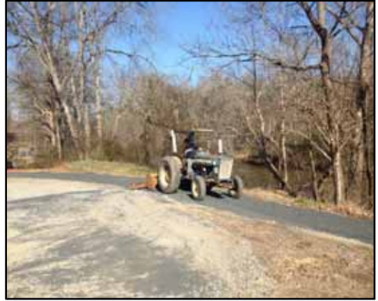
P2 – Grading new trail surface in Randleman
