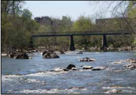
P1 – View of pedestrian bridge from Franklinville to Faith Rock (Credit:Town of Franklinville)
