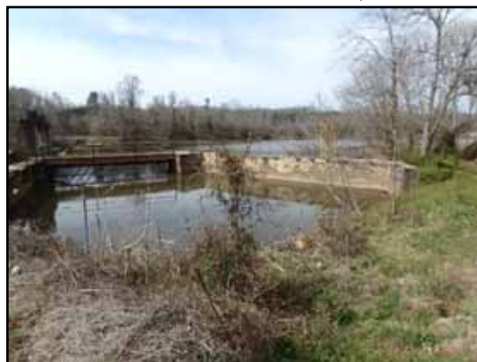
P6 – View of active Franklinville Upper Dam
