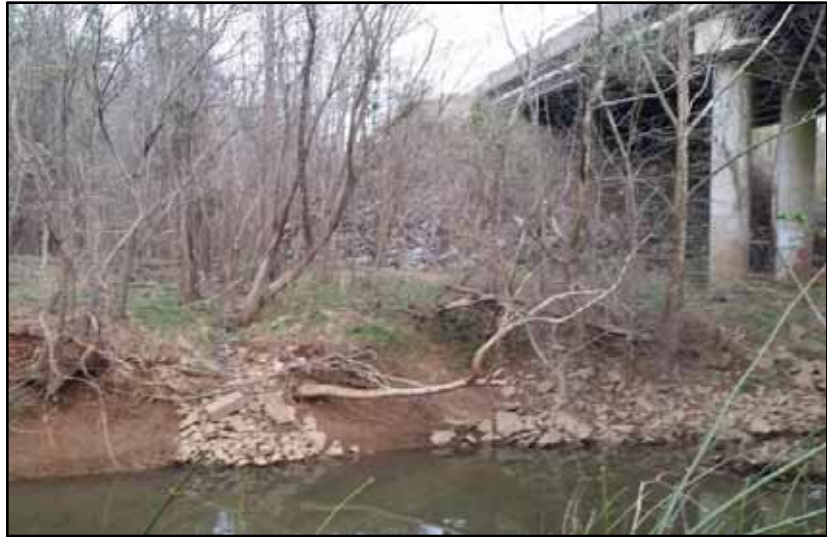
Photo 5: Sandy Creek Crossing with US 64 Bridge Above Credit: Town of Franklinville
