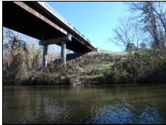
P6 – Old Liberty Road bridge over Deep River
