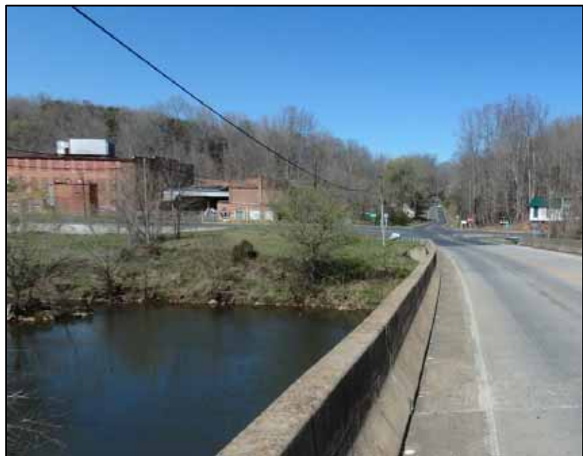
Photo 6: View of Cedar Falls Closed Mill from Bridge over Deep River
