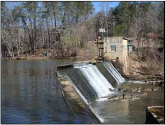
P3 – Cox's Dam
